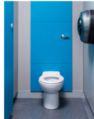
Education: Installed at Broom Valley Community School
