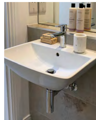
Residential: Installed at Derwent Walk
