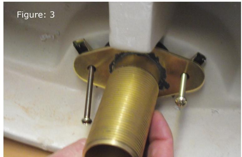
Figure 3: Using fixing bolts and butterfly clips screw waste fixing to basin.
