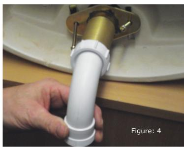
Figure 4: Fasten waste connector on to waste outlet.
